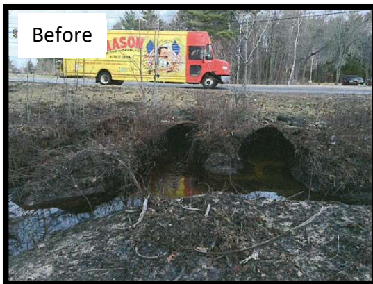
Sample 319 grant project: Triple-barrel culvert causing bank erosion and impeding fish passage was replaced with a 16' pre-cast concrete bridge.
