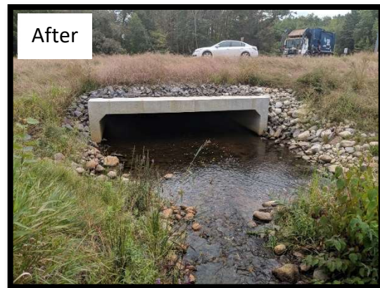
Sample 319 grant project: Triple-barrel culvert causing bank erosion and impeding fish passage was replaced with a 16' pre-cast concrete bridge.
