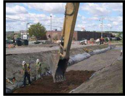
Watershed-based plan implementation - installation of bioretention swale.
